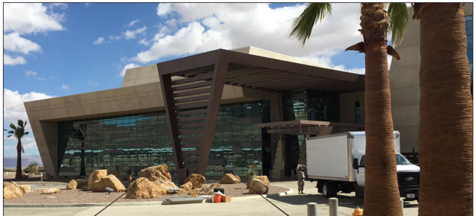
TOP: A view of the main entrance to the 947,000-square-foot, $500 million state-of-the-art Carl R. Darnall Army Medical Center at Fort Hood, Texas, which opened in 2016.
